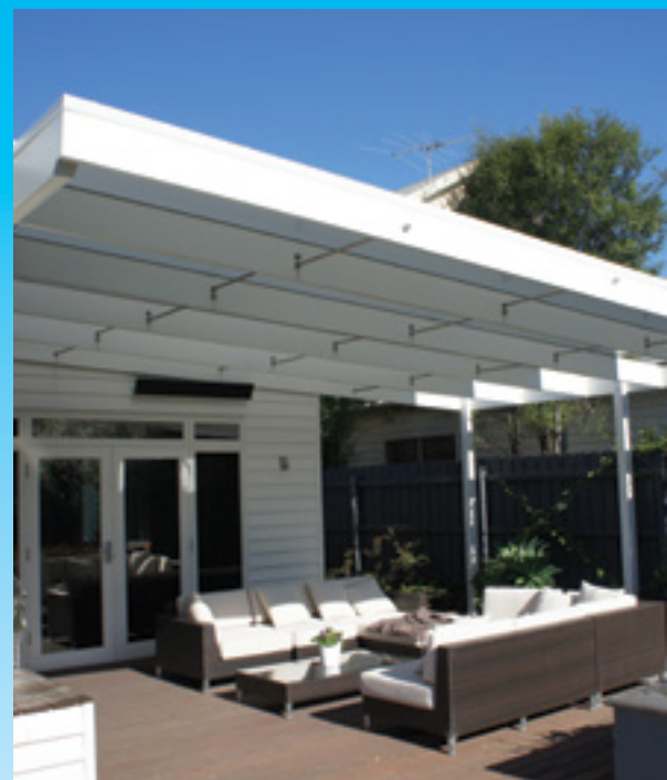
Posts and beams
